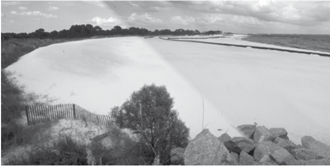
Figure 3. Beach nourishment activities along the channel shoreline occurred over July/August 2003. Black plastic piping that was used to transport quartz sand to the beach is visible in the background.
