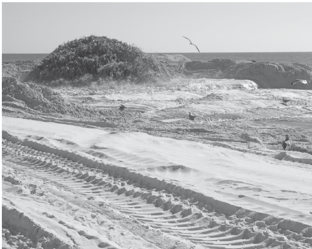
Figure 2. Active beach nourishment along Panama City Beach, Florida. The image is from January 2006, and shows the manner in which the sand-water slurry is pumped onto the beach. The water drains leaving sand deposited under energetic aqueous conditions. The water-sand plume is approximately 2.5 m high.
