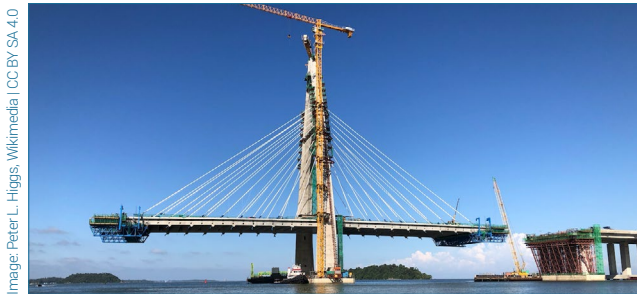
Figure 4. A cable stay bridge under construction
